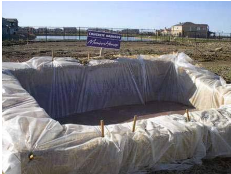
Plate 2.1: Typical Temporary Concrete Washout Area
